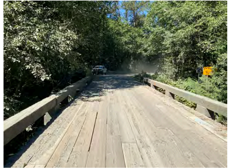
Approach from Right Bank when facing downstream
