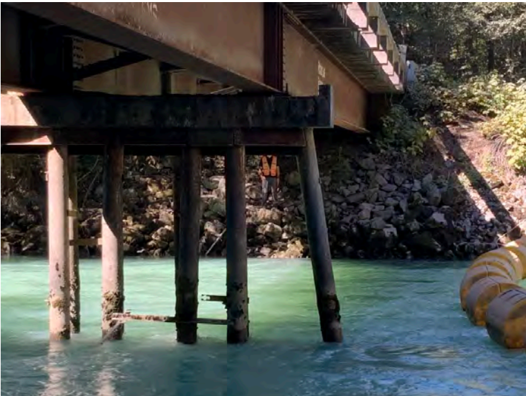
Right Bank Abutment when facing downstream
