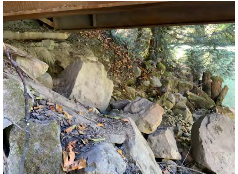
Left Bank Abutment when facing downstream
